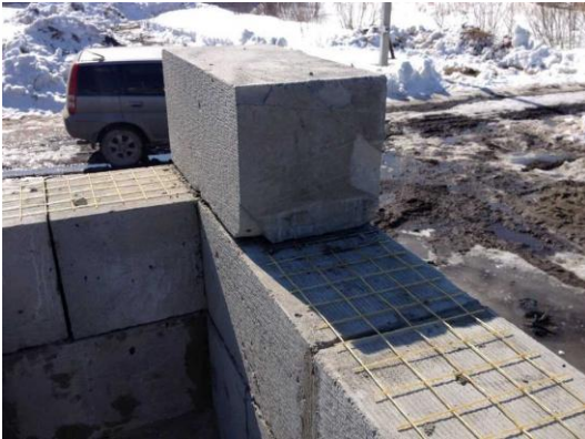
Masonry reinforcement
