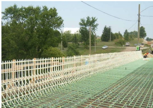
Reinforcement of bridges
